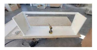
4) Lay one of the panels with the slots facing up and align face and sides panels to top of the panel.
